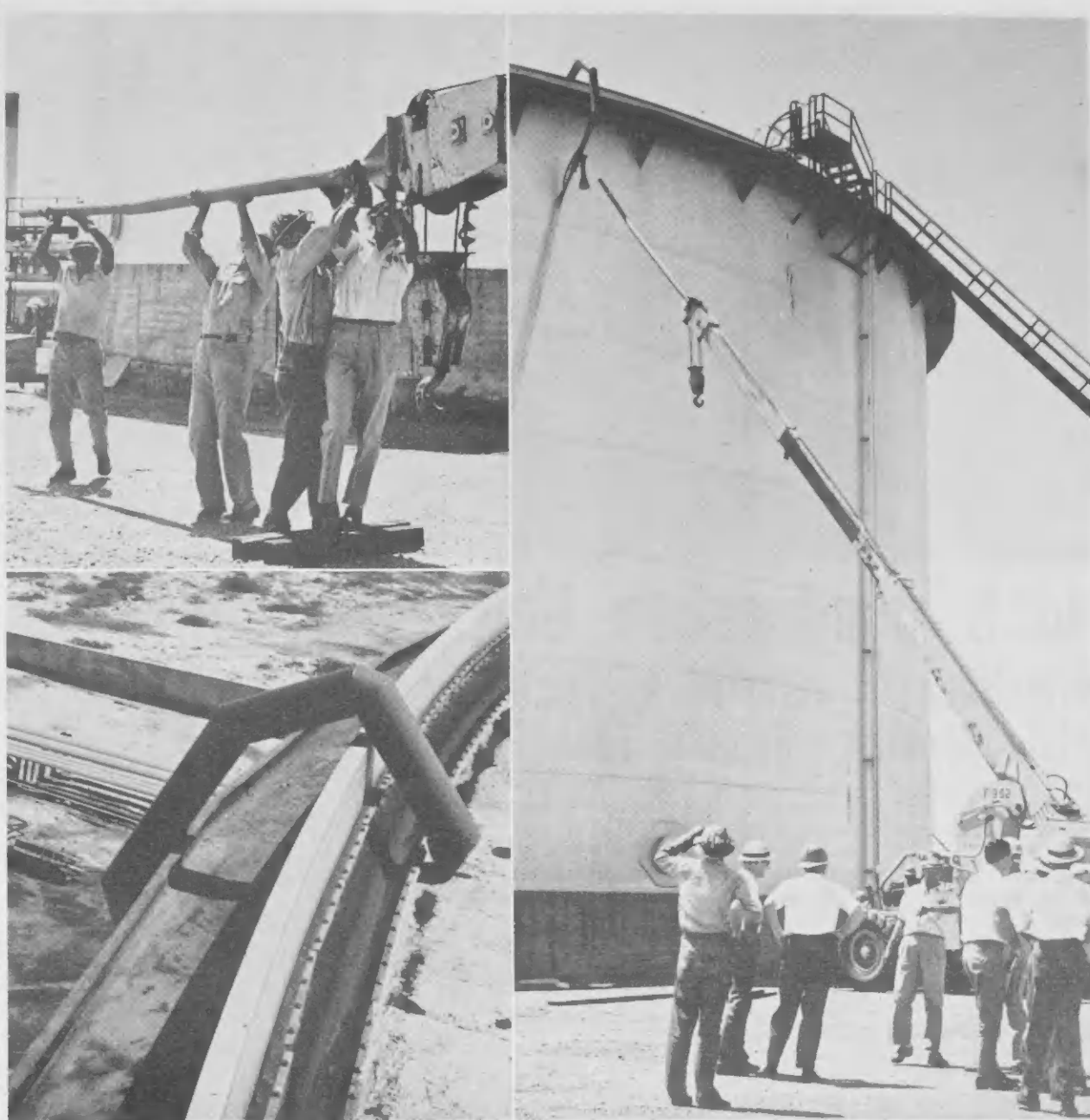
NEW WAY to reach the tops of the tallest tanks in firefighting drills is demonstrated by this attachment, den exercicio pa paga candela ta demonstrá pa medio fitted on a hydraulic crane. It allows quick placing of a di e adición aki, cual ta instalá ariba un grua hidráulico. Esaki ta permiti pa pone un tubo di spuit cu curva gooseneck foam outlet over the lip of this tank, sixty pa foma it rapidamente pa pasa ariba e rand di e tanki, six feet above the level of the ground.
